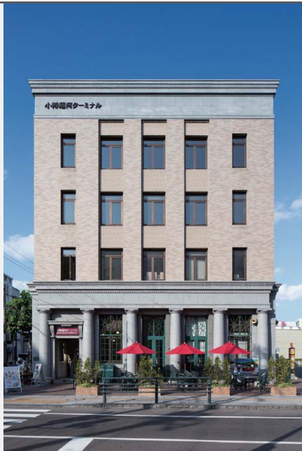
Location:1-12 Ironai 1-chome, Otaru Built:1922(Taisho11) Structure: 4 story reinforced concrete building
