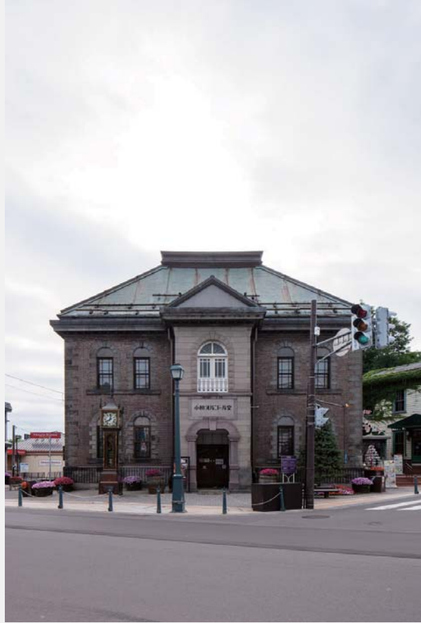
Location:4-1 Sumiyoshi-cho, Otaru Built:1912(Meiji 45) Structure: 2 story timber framed brick building
